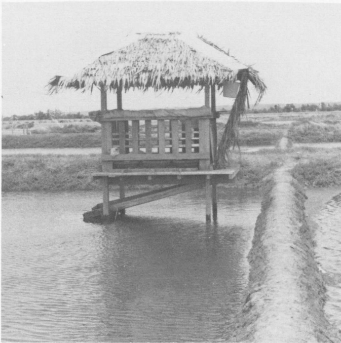
Pig pen built over fishpond as part of experiment in pig-fish combination culture at the BAC. Pig manure and uneaten feed washed into the pond daily provide food for the fish and fertilization for the pond.
