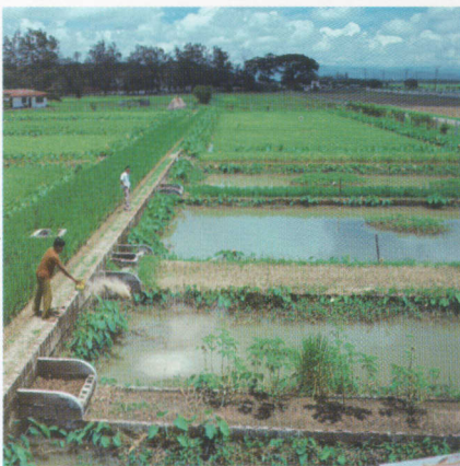
Rural development: The Center assists with the design, construction and management of aquacultural research facilities as shown in this fish-rice-vegetable facility in the Philippines.
