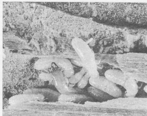
Subterranean termite infestation.
