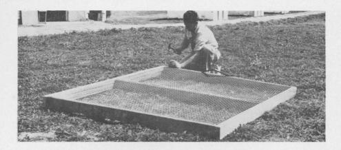
Base of the shelter is 6 feet wide and 8 feet long. It is formed by placing four 2-by-4's on edge, and by nailing ends of 8-foot pieces to the two 6-foot lengths. A third 6-foot 2-by-4 is placed halfway between the ends. This center brace is
