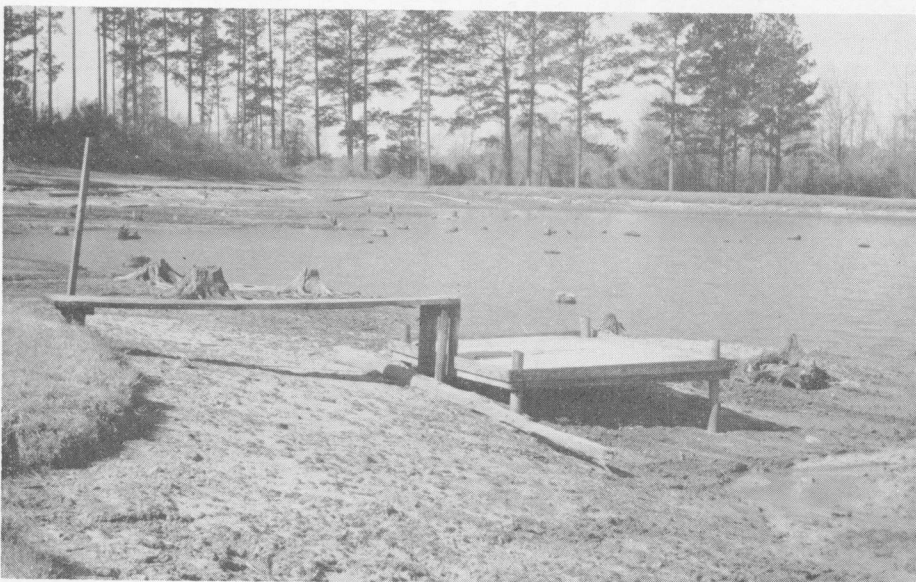
A single platform can be used to fertilize up to 15 acres of water. Here the pond has been drawn down to show construction details. Fertilizer is placed on top of platform, which is 1 ft. under water when pond is full.
