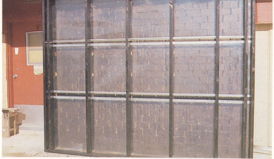
FIG. 1. This solar collector, made of stacked solid concrete blocks with a surface of two layers of fiberglass material, offers limited storage capabilities.
