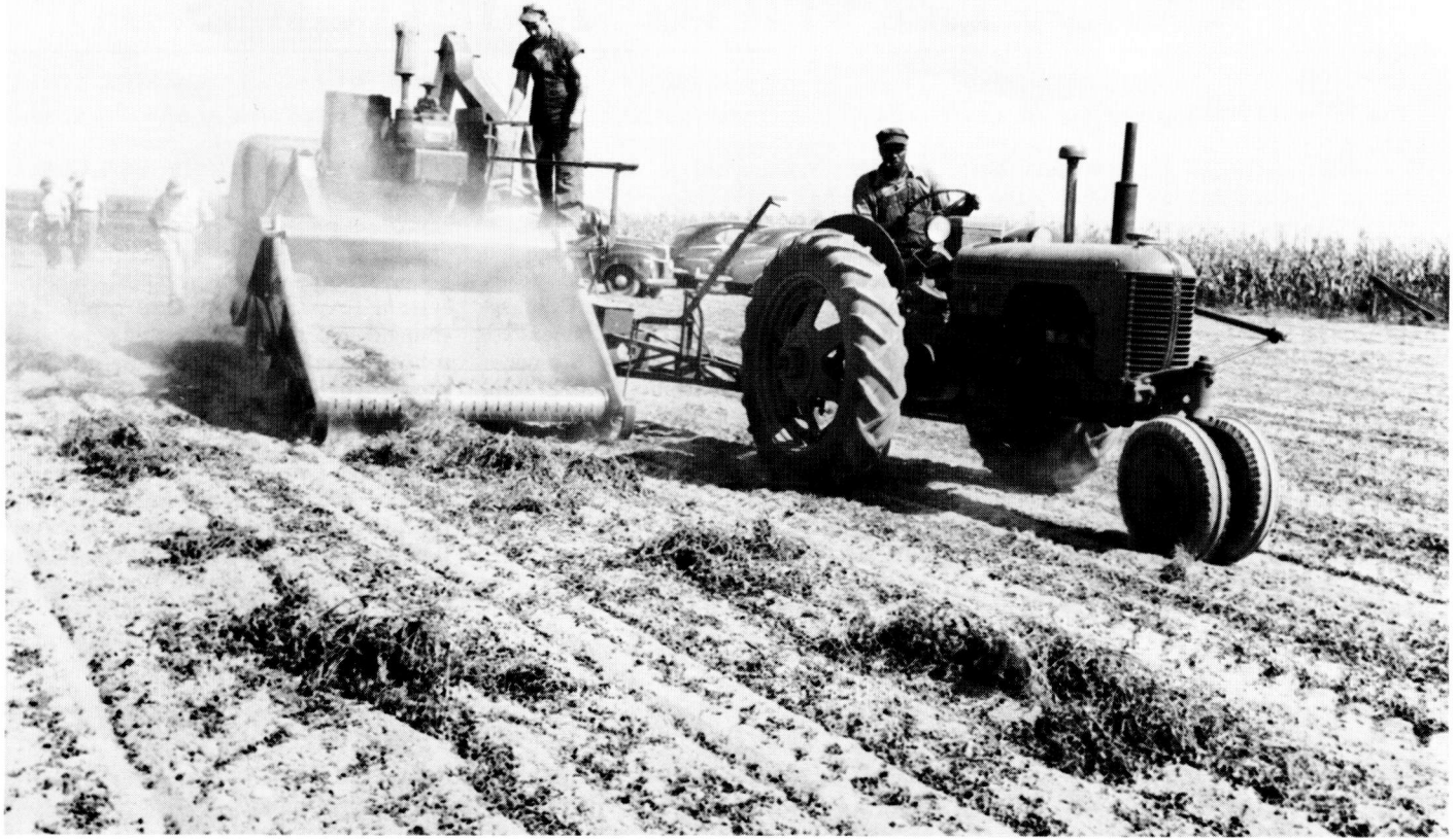
Cooperative work between the Experiment Station and industry led to development of mechanical harvesting methods for peanuts.
