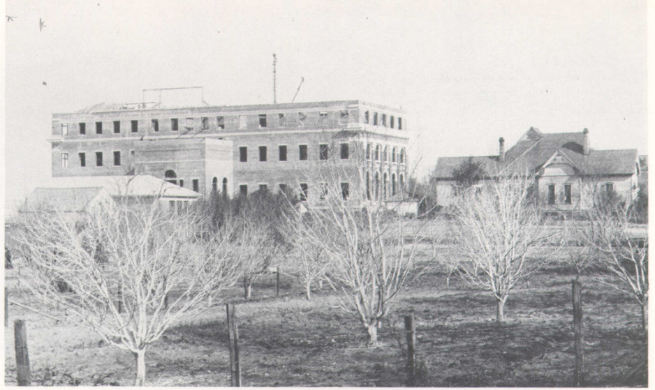
Comer Hall under construction in 1907. It burned in 1920, but was rebuilt and still presides over Ag Hill.
