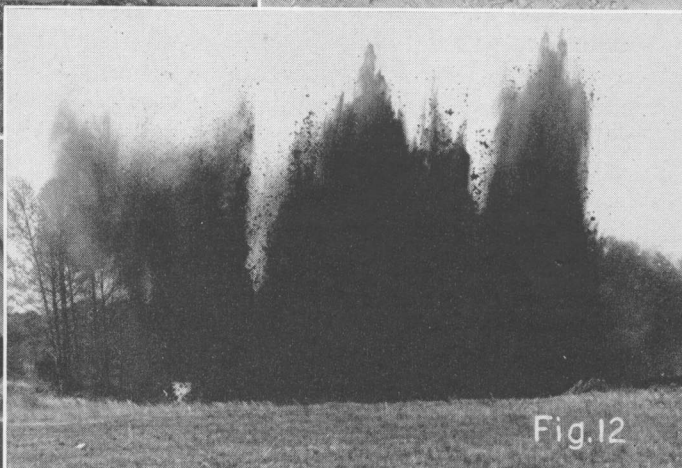
FIGURE 9. Guide stakes are set along center of core preparatory to setting dynamite. FIGURE 10. Close-up of method of punching holes and inserting sticks of ditching dynamite. FIGURE 11. Electric cap is inserted in hole punched in side of dynamite stick. This hole should be about 3 inches deep and one-half inch in diameter. FIGURE 12. Cap is ignited and entire line of dynamite is exploded. Note the height to which mud and dirt are thrown. Since most of this material falls outside of trench, no one should be nearer than 500 feet.
