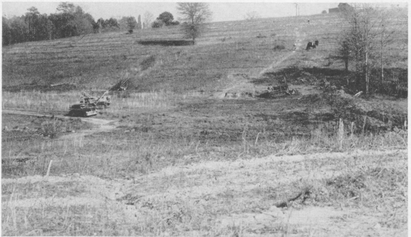
FIGURE 2. Tractors and teams are used to remove the trees, brush, and ground litter from a dam site in preparation for marking off the base of the dam.
