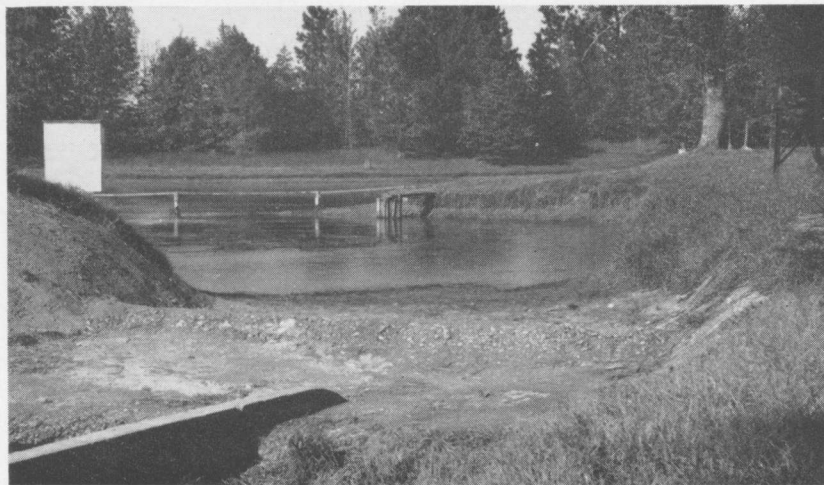
FIGURE 34. This concrete spillway for a 1.3-acre pond has a low wall across it to obtain desired water level in the pond. The entire floor is paved to prevent erosion and end of dam is faced with concrete to prevent flood water damage.
