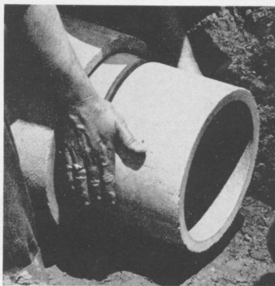
FIG. 17. Asbestos-cement pipe, rubber, rings, and collar used to assemble joint.
