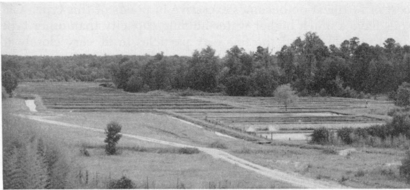
FIGURE 1. A relatively flat, gently sloping area with a tight clay subsoil makes an ideal location for construction of a hatchery.
