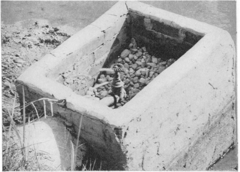
FIGURE 11. A gravel filter similar to the one above should be used to prevent the entry of wild fish into minnow ponds. The filter must be periodically cleaned to maintain its effectiveness.
