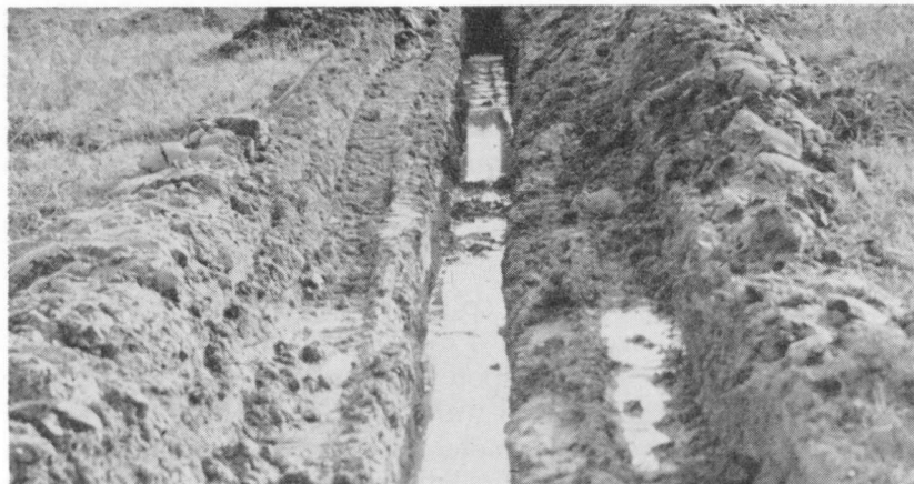
FIGURE 3. The base for the dams should be excavated with a tractor down into an impervious layer of clay to form a water-tight seal between the bottom and sides of the pond.
