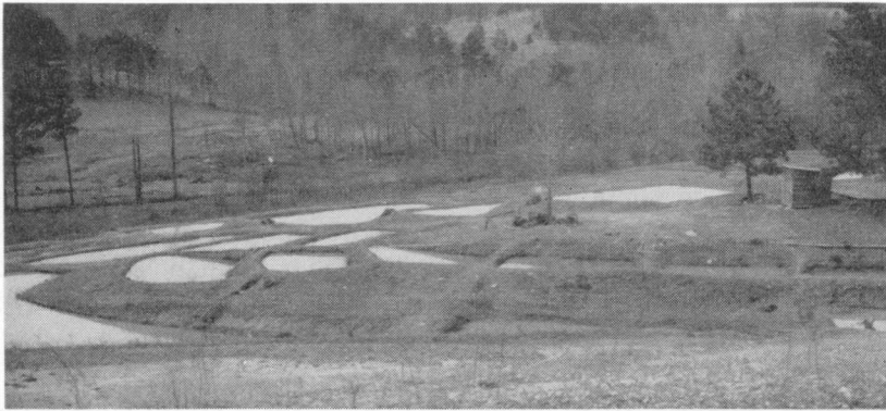
FIGURE 2. Where the soil is sufficiently water-tight, ponds can be located on hillsides in a terrace-like pattern.
