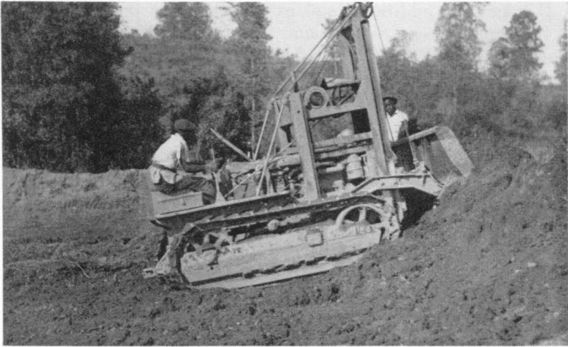
FIGURE 4. When a bulldozer is used to push up the dams, the dirt can be packed sufficiently by running the tractor up and down the sides and on top of the fill.
