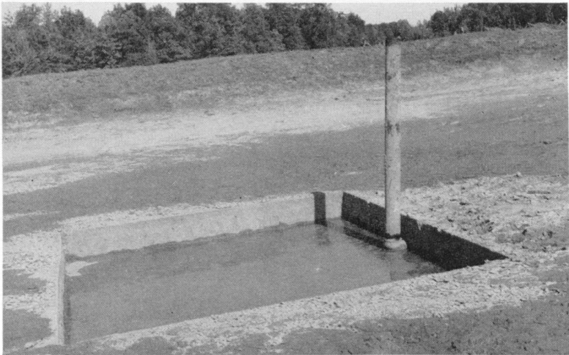
FIGURE 7. A catch basin about 12" deep and 10'-0" to 15'-0" square facilitates the harvest of minnows when the pond is drained.
