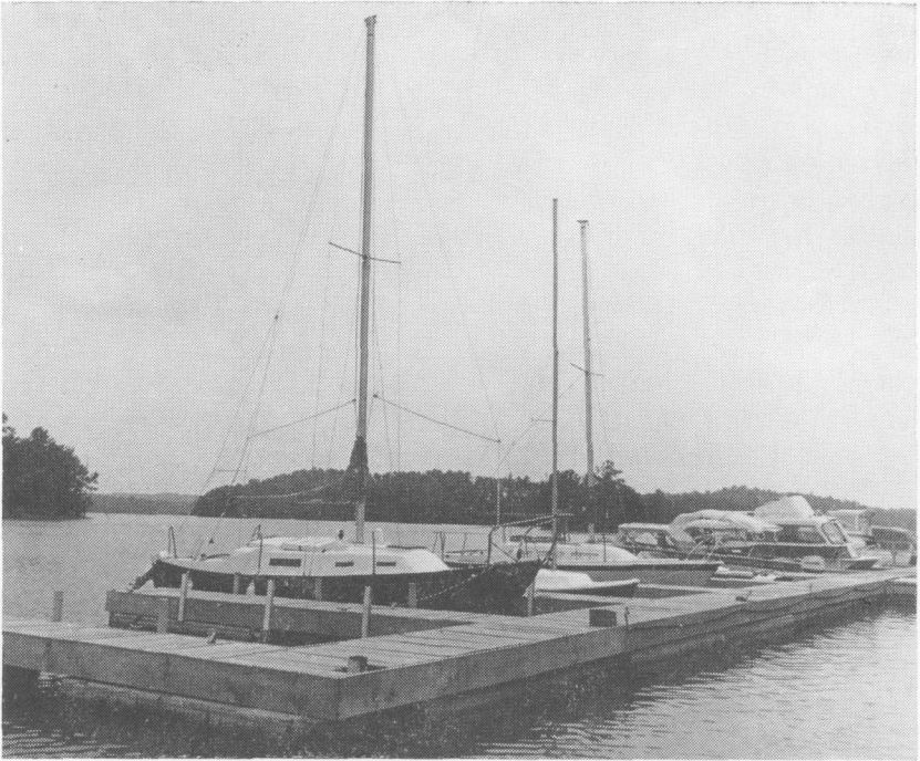
FIG. 6. Floating docks were used on lakes where water level fluctuated widely.
