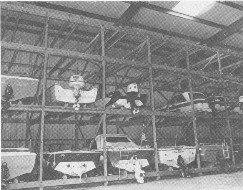
FIG. 7. Warehouse-type storage sheds were more expensive to build but owners reported lower maintenance costs for this type facility.
