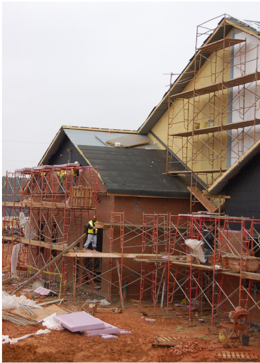
ANOTHER BRICK IN THE WALL —Workers brick up the front of the new laboratory building at Shell Research Center. The laboratory will provide a great deal more space for research and study.
