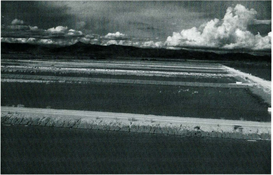
Figure 11. Levee containers used in the production of shrimp in Honduras, South America.
