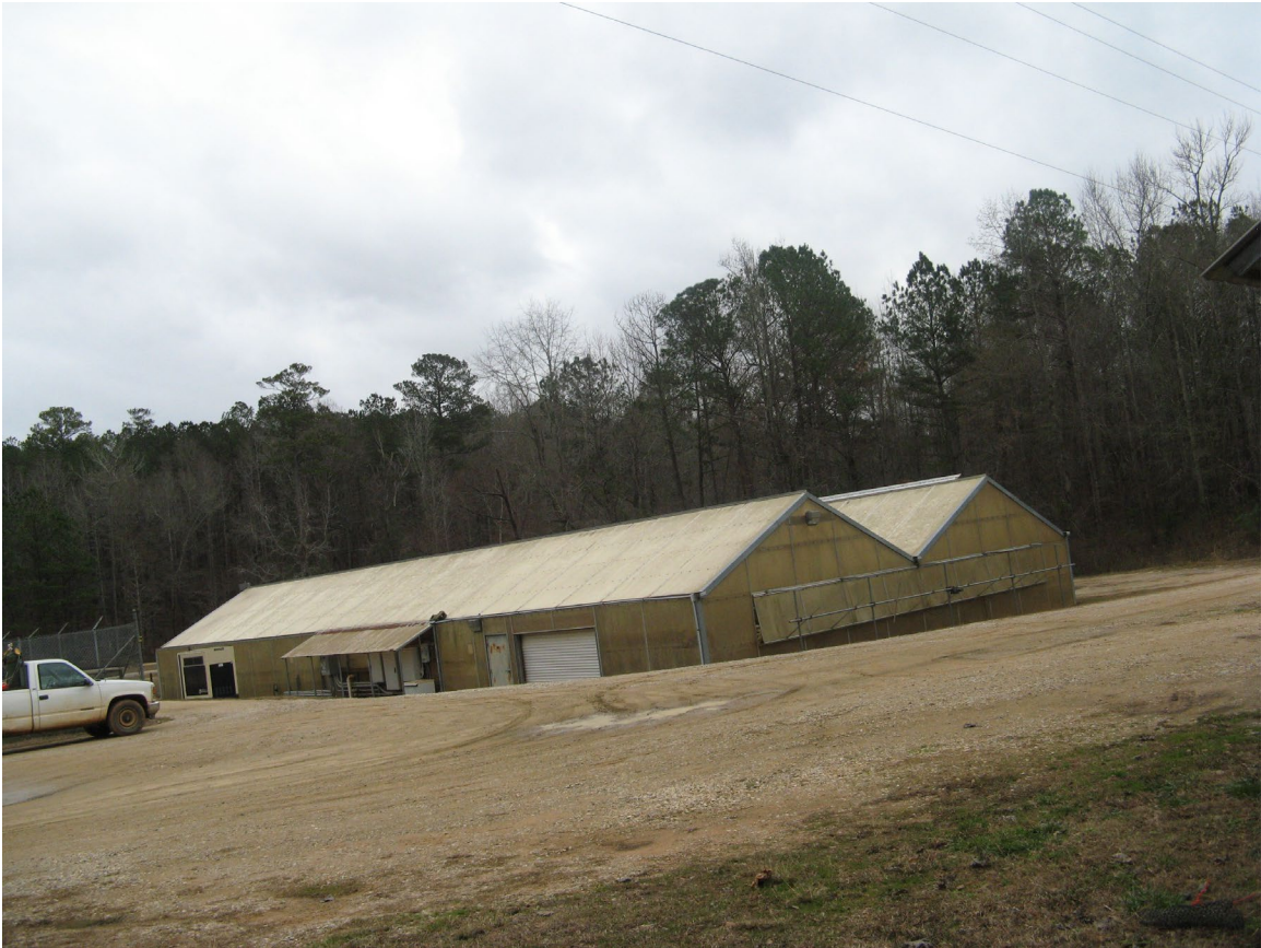
Figure 77. The genetics hatchery and holding facility. Part of it was completed in 1991. It was renovated and expanded in 2009.
