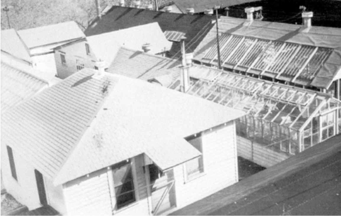
Figure 16. Much of the Swingle and Smith research on the evaluation of inorganic fertilizers in the production of plankton in glassware containers was conducted in these greenhouses. They were located directly behind Comer Hall.
