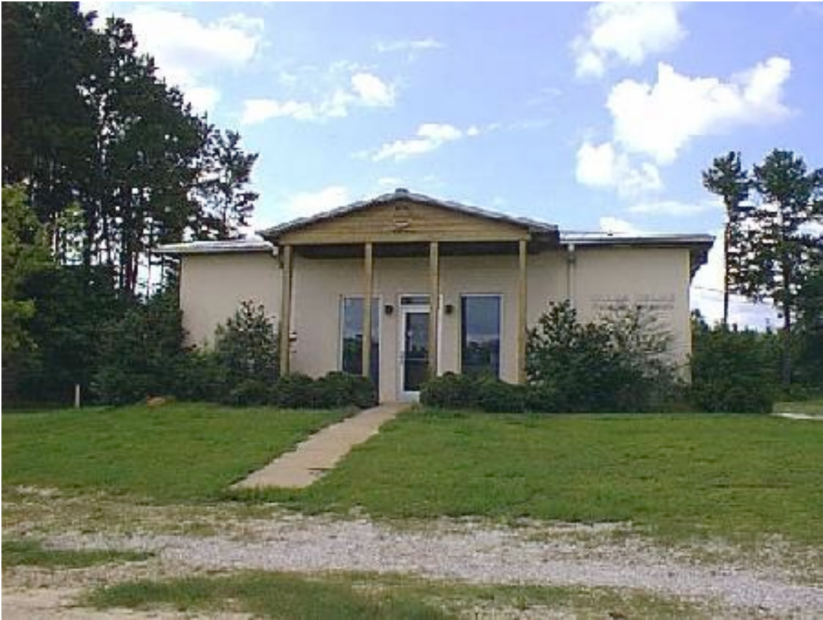
Figure 74. View of the Ireland Center. Over the years, several additional structures have been constructed around the north side of the main building as our extramural program in fish management in 'public' waters has expanded.
