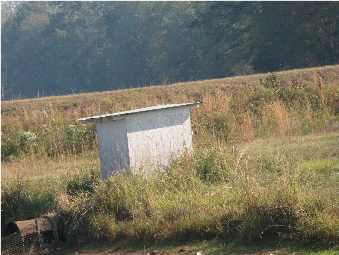
Figure 85. Pump-house at the eastern end of Pond S-8. Activating the pump lifted water over the 'divide' between the Swingle Creek and Funchess Creek Watersheds. Note the south end of the Pond S-14 dam in the background.
