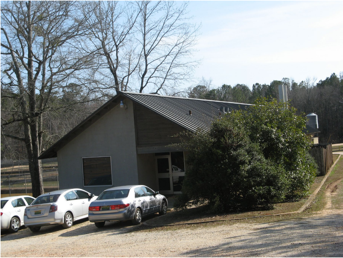
Figure 76. Genetics and Breeding Laboratory Building. Building was constructed with funds provided by the Mellon Foundation. It is located just south of County Highway 072 on the north end of the Soughahatchee Farm. It was completed under contract in 1990.
