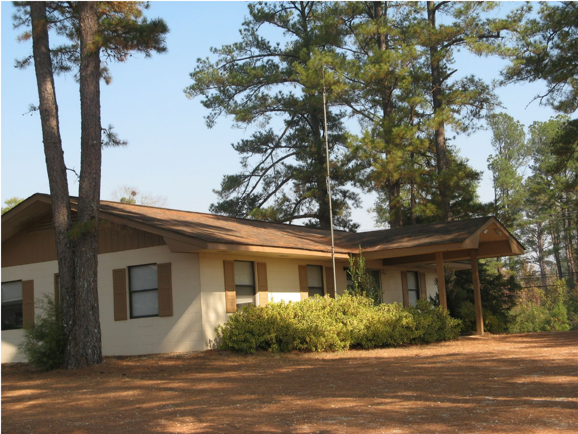
Figure 75. Field Operations Headquarters Building. Completed on the Soughatchee Farm in 1990.
