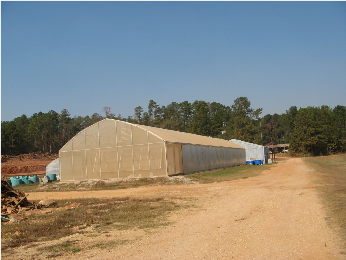
Figure 107. Hydroponics laboratory on the Soughahatchee Farm. Building is located just south of the Fish Processing and Technology Laboratory.
