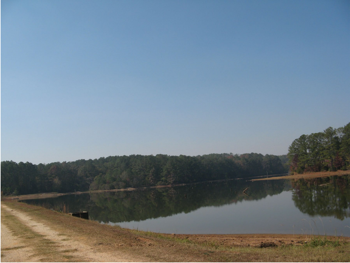
Figure 58. View of Farm Pond 11 from the southeast. Note the 4-foot water outlet in the lower left-hand corner.
