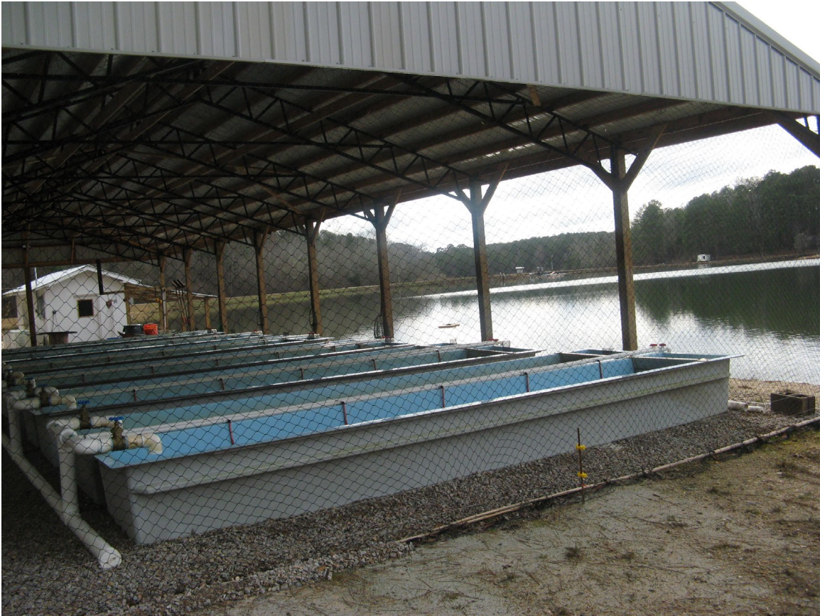
Figure 66D. Pole barn erected of the east side of Pond S-1 in 2017. It is to Be used by the Peatman Work Group. It protects a series of large plastic troughs. The Pond S-1 dam is at the center right. Note that the 'ticket shed' used in research on the sale of fishing privileges is shown on the left margin of the Figure.
