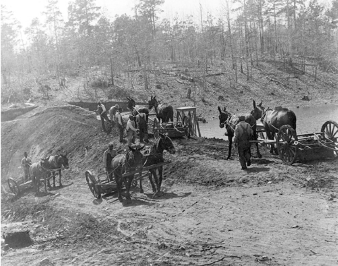
Figure 6. Mules and slip-scrapes constructing the dam for Farm Pond 1.
