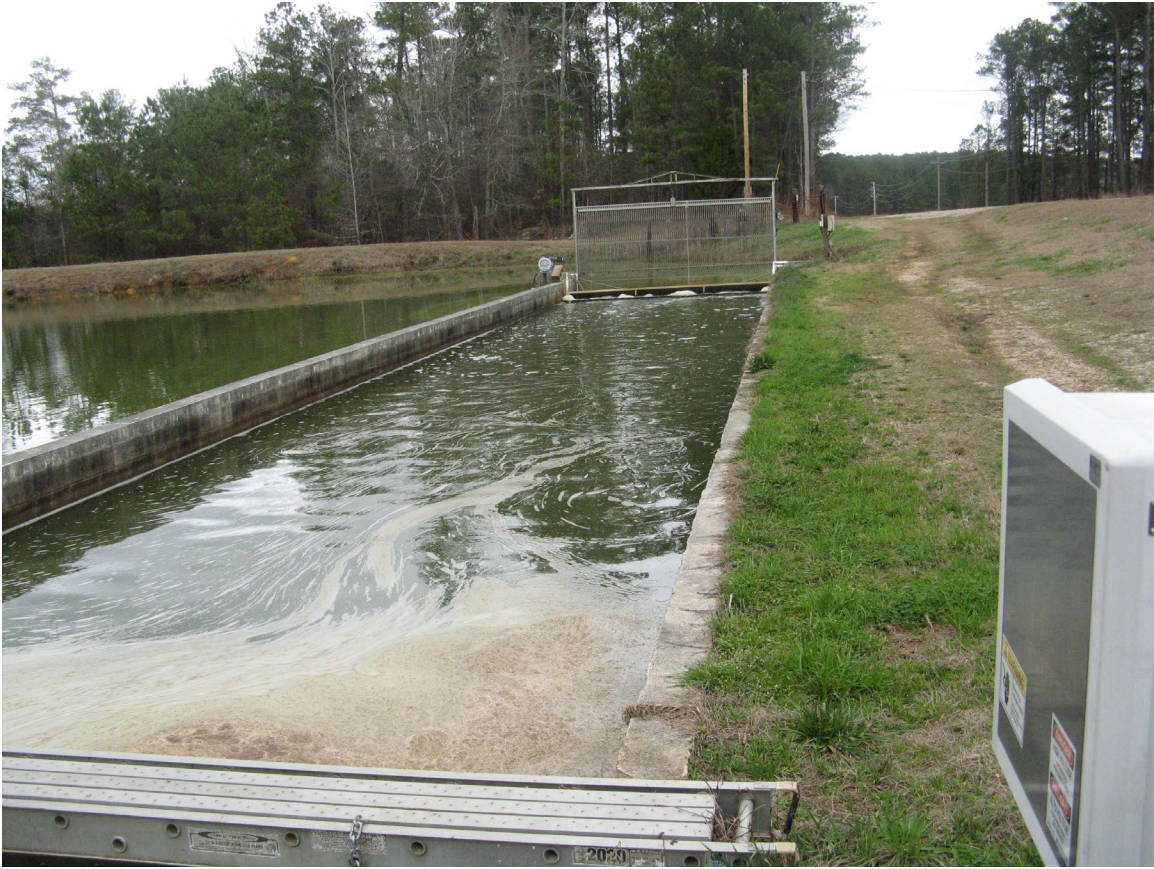
Figure 108. 'Fixed' production raceway constructed in Pond S-10 (a 'terrace-water' pond) on the Story Farm (Figure 18C). Raceway was constructed in 2005 to facilitate fish harvest. It was converted to a production raceway in 2016.
