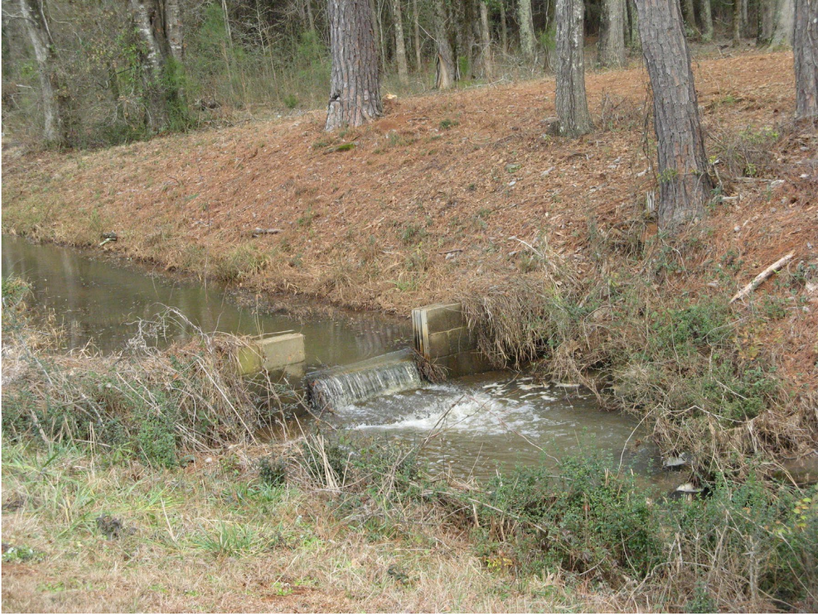
Figure 84A. Low dam on the Diversion Ditch at Pond S-6. By placing a board in this dam, a small reservoir is created upstream. A pipe installed in the reservoir carries water by gravity overland to Pond S-8.
