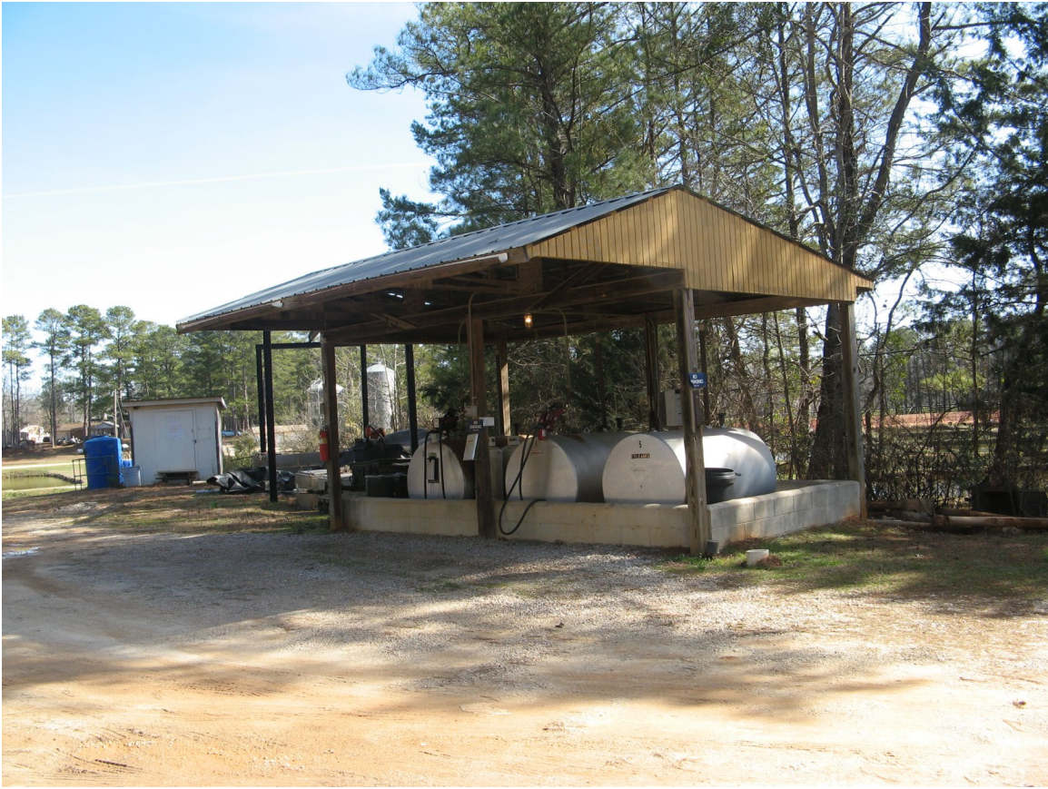
Figure 65. Fuel storage facility on the Soughahatchee Farm. Note that the small chemical storage building is located near the left-hand margin of the picture.
