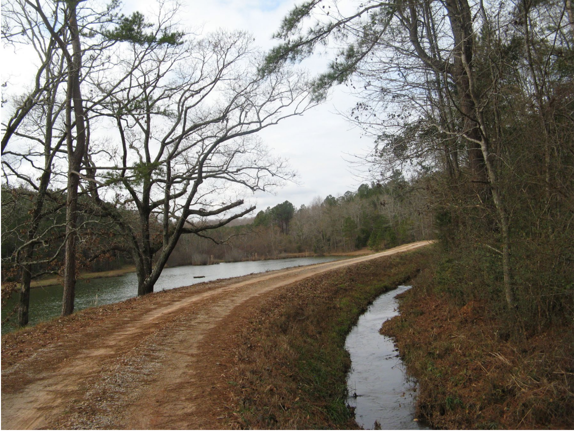
Figure 18E. Diversion ditch east of Pond S-6. Construction was initiated in 1947. The 'upper' end of Pond S-6 is in the background.
