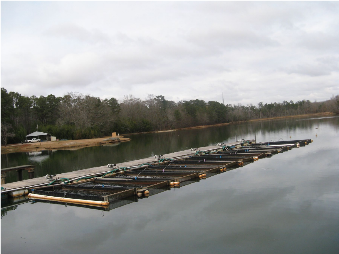
Figure 79A. Floating research containers installed in Pond S-1. These were installed for use of the Peatman Work Group.
