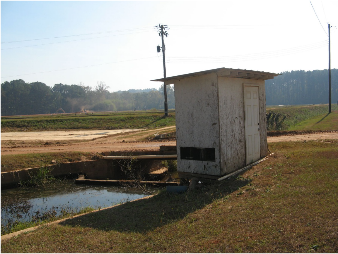
Figure 84. Pump-house on Funchess Creek adjacent to the site of the demolished 'Counting Shed.' By activating the pump, water flowing down the Creek could be returned to the 'Closed System.'
