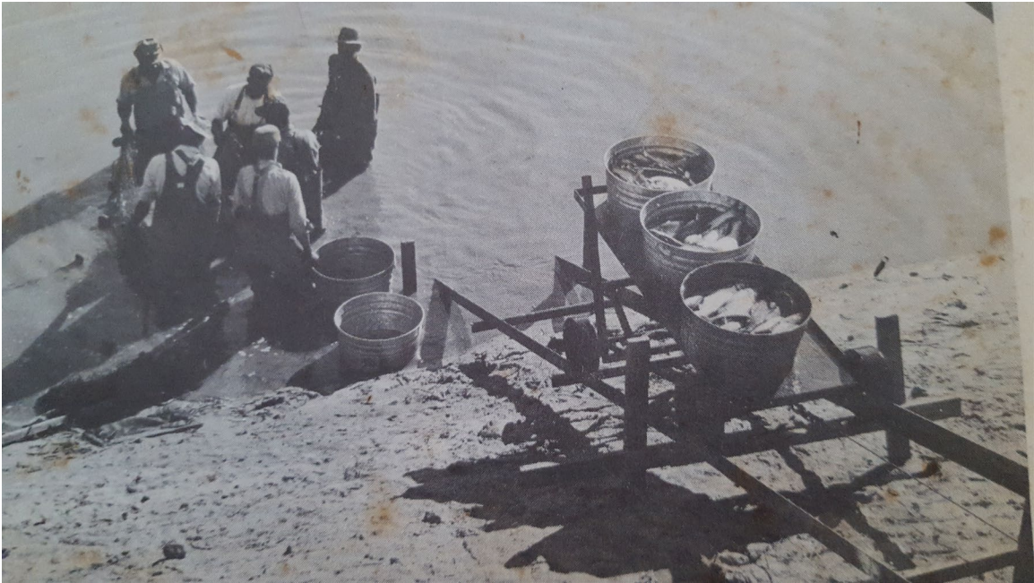
Figure 50. 'Track' arrangement for lifting 'tubs' of fish from the 'containment' area in the draining pond to the hauling truck on the dam above.
