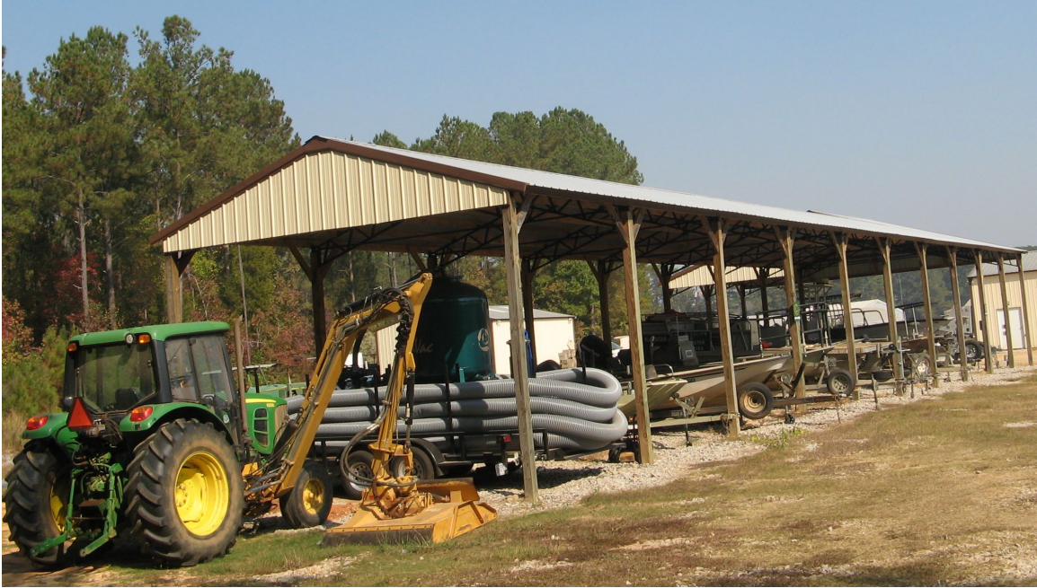
Figure 66. Boat and tractor storage shed. It is located in the southwestern boundary area of the Soughahatchee Farm. Construction completed in 2009.
