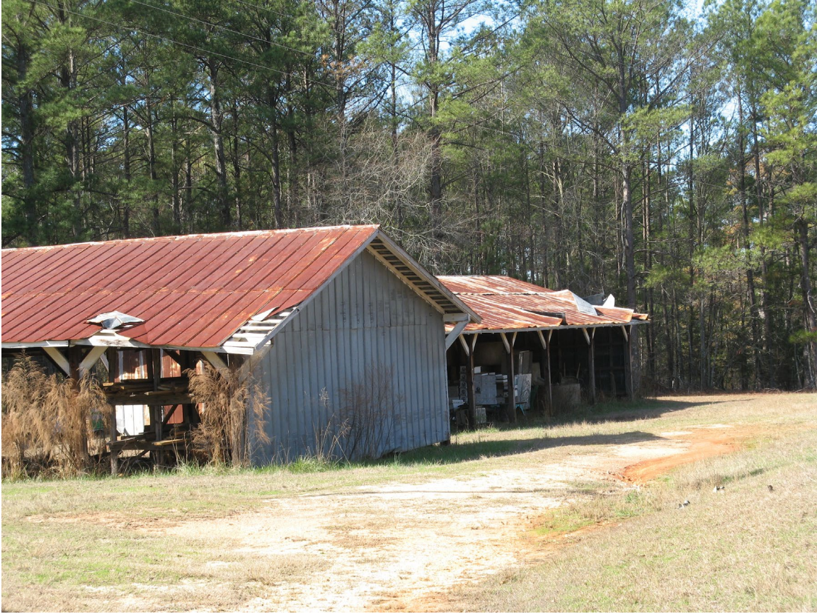
Figure 62. Two of the 'Field Storage' buildings constructed at the rear of the old Field Headquarters Site on the Story Farm.
