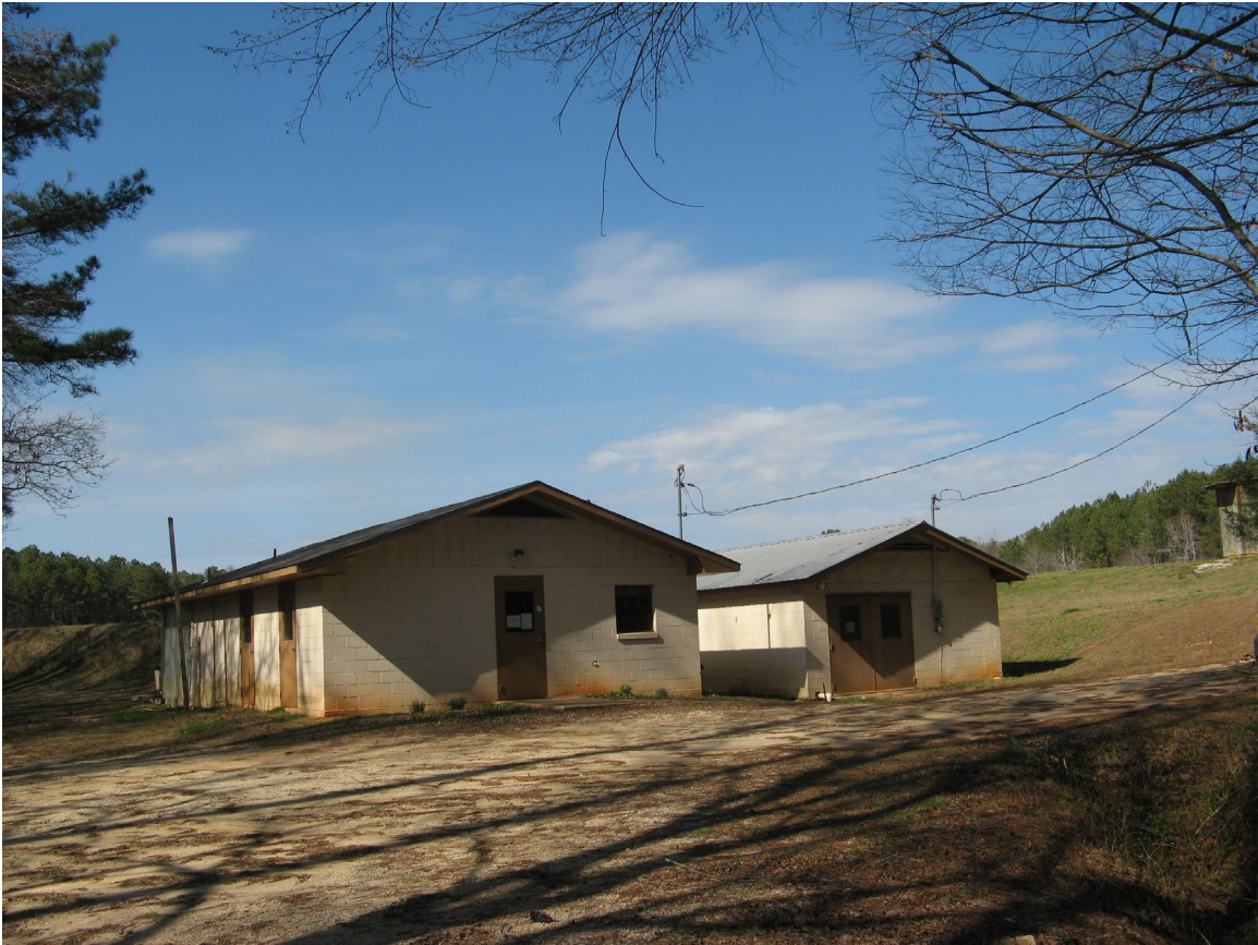
Figure 79. Fish Health Laboratory, located below the east end of Pond S-6 dam.
