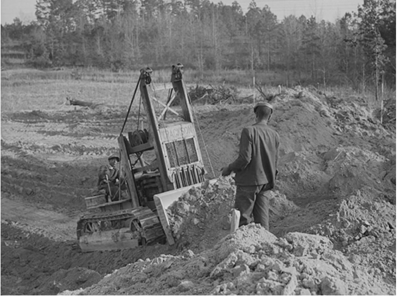
Figure 31. Bo Tarver 'pushing-up' dam on Farm Pond 6 using the 'Funchess' bulldozer.
