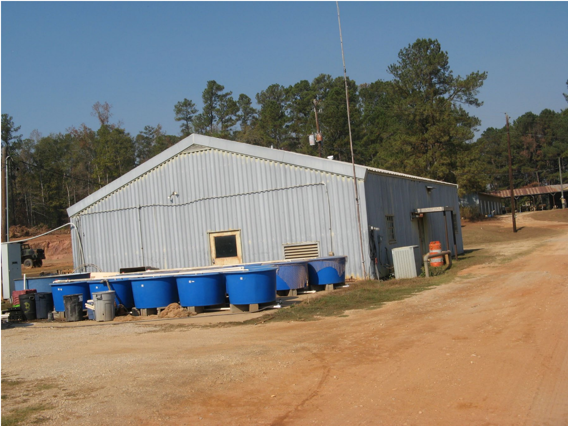
Figure 72. Fish Processing and Technology Laboratory. Constructed under contract in 1975.
