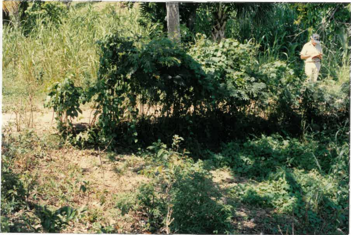
This picture shows the checkdam from a downhill position. The amount of soil accumulated can be appreciated by noting the difference in the level of the roadbed and the slope of the soil at the base of the checkdam (in shadow).
