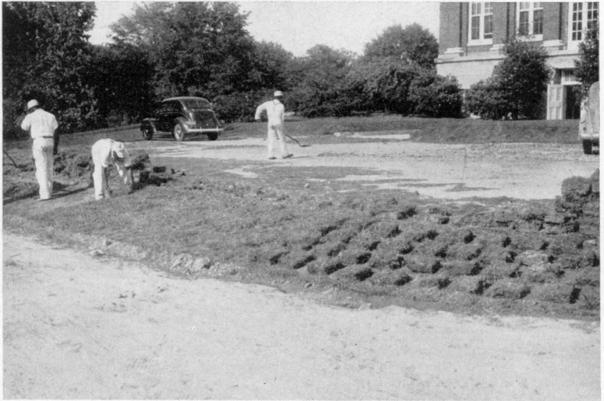
Sodding an area solid with blocks of Bermuda grass sod. On the right the blocks of sod may be seen while on the left the area has been sodded by placing the blocks in place.
