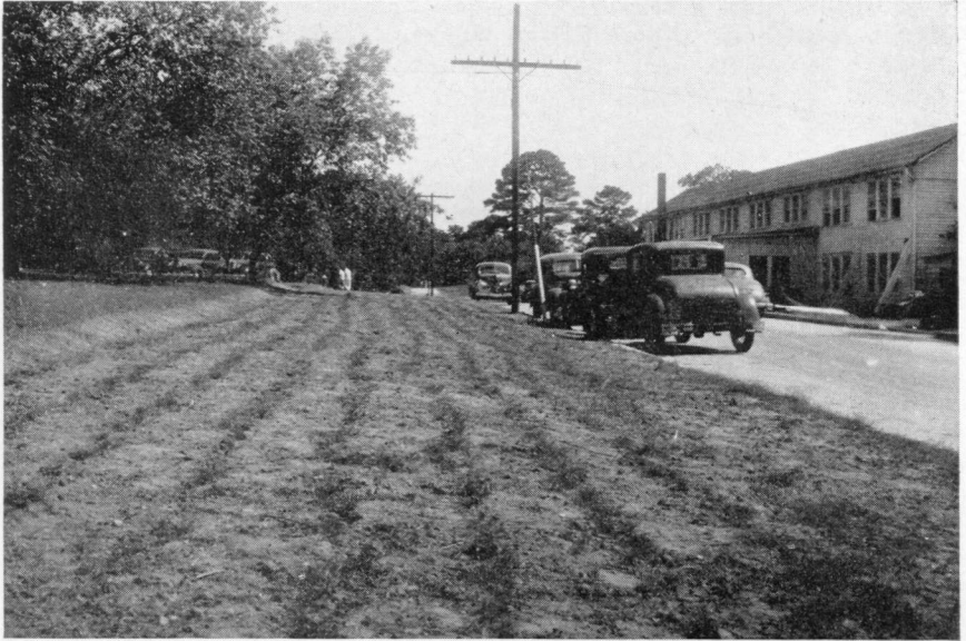
An area that was strip sodded with Bermuda grass. Note the rows run on the contour to check washing.
